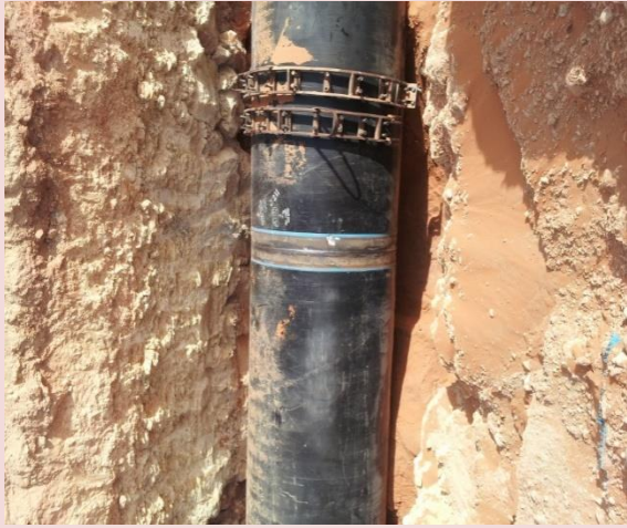
PIPE LINE INSTALLATION 96"OD. & 72" OD
