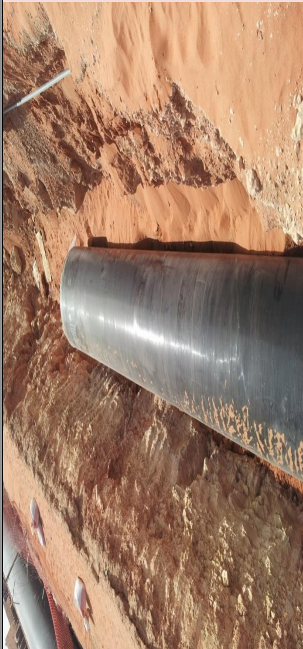
PIPE LINE INSTALLATION 96"OD. & 72" OD
