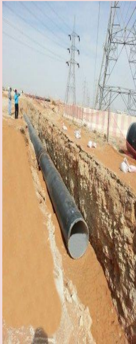
PIPE LINE INSTALLATION 96"OD. & 72" OD
